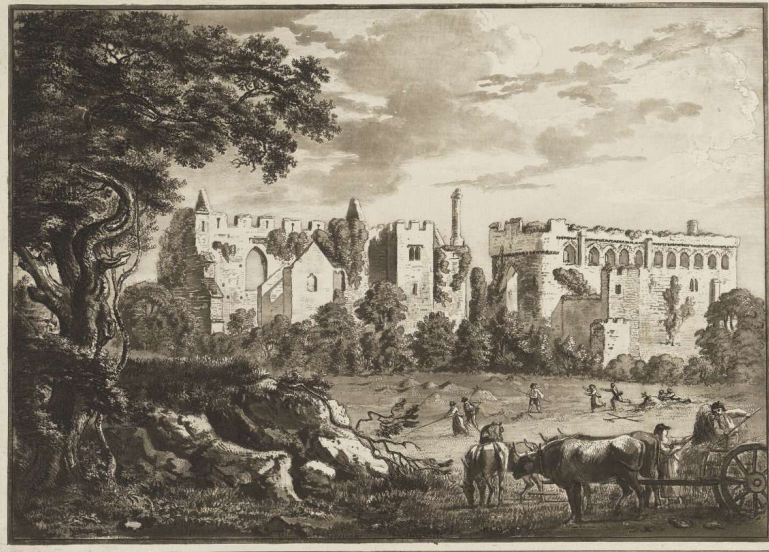
Part of the Remains of Llanphor, near Pembroke.
