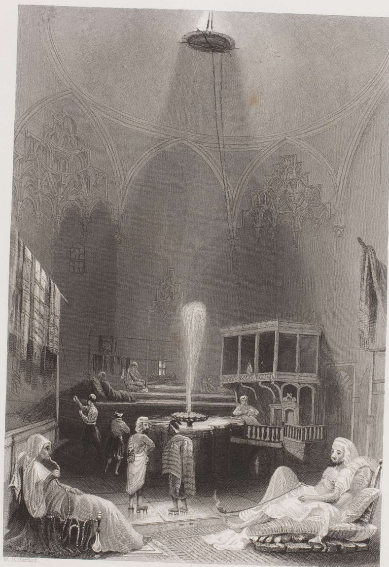
COOLING ROOM OF A HAMMAM.
